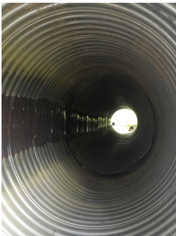
Looking upstream through culvert
